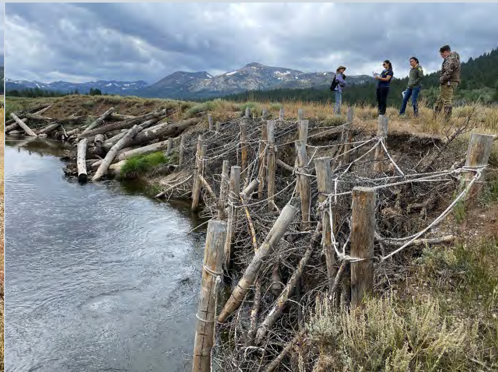
Site 2 had some extensive damage due to high flows
